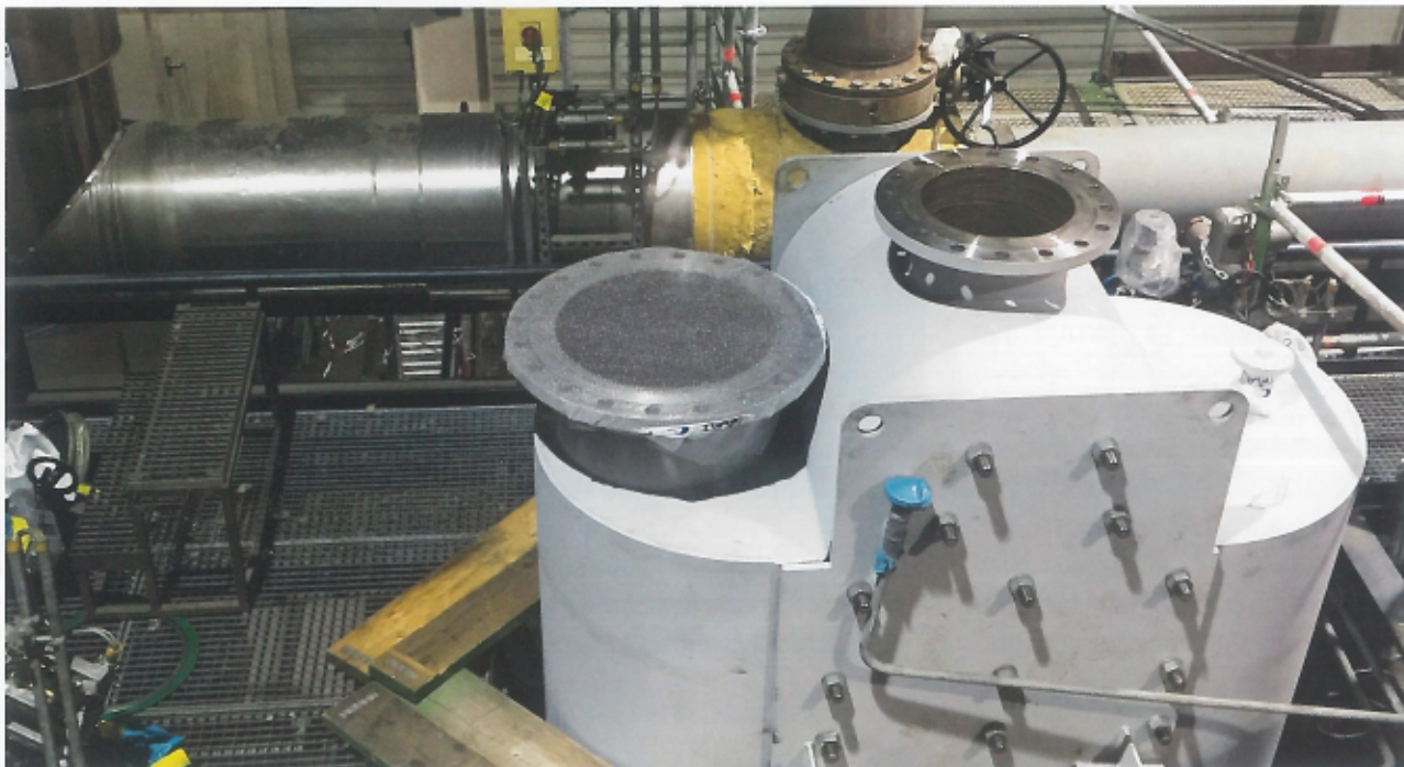
Installed Hybrid tubular heat exchanger for hot water preparation in combined heat and power plants
